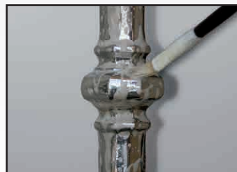
Applicazione del derugginante E4051/D deve coprire tutte le parti inquinate Application of the de-rusting product E4051/D: all polluted parts must be covered
